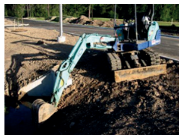
Excavation of pits
